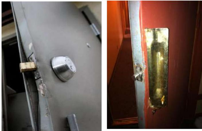
*-Small latch guards and unprotected doors are vulnerable to being pried open or damaged beyond repair and offer little to no security.*
