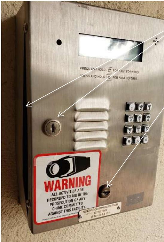
*-Telephone Entry Systems are usually constructed of thin gauge steel and a low security cam-lock. When left unprotected, these boxes can be easily pried open.*
